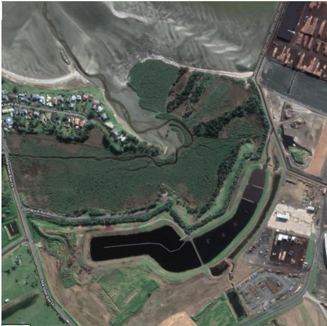
Figure 7 - Aerial View of the Stormwater Ponds circa 2018
